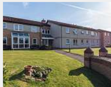
Above: Sidey replacement project.
