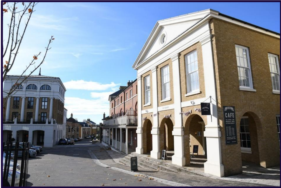
Figure 23: Examples of the architectural style of Poundbury drawing heavily on traditional British styles, including Georgian, Regency, and local Dorset vernacular
