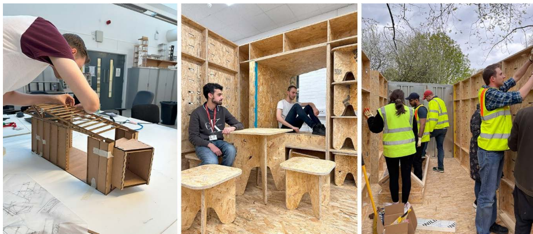
Fig. 5. Ivett and Stefanescu. The Ripple Effect: detailing through sketches and models, fabricating all components using the waterjet cutter by the Master of Architecture students, and the on-site installation of the Pop Up in Lomeshaye Park. 2023-2024. Source: Author's own.
