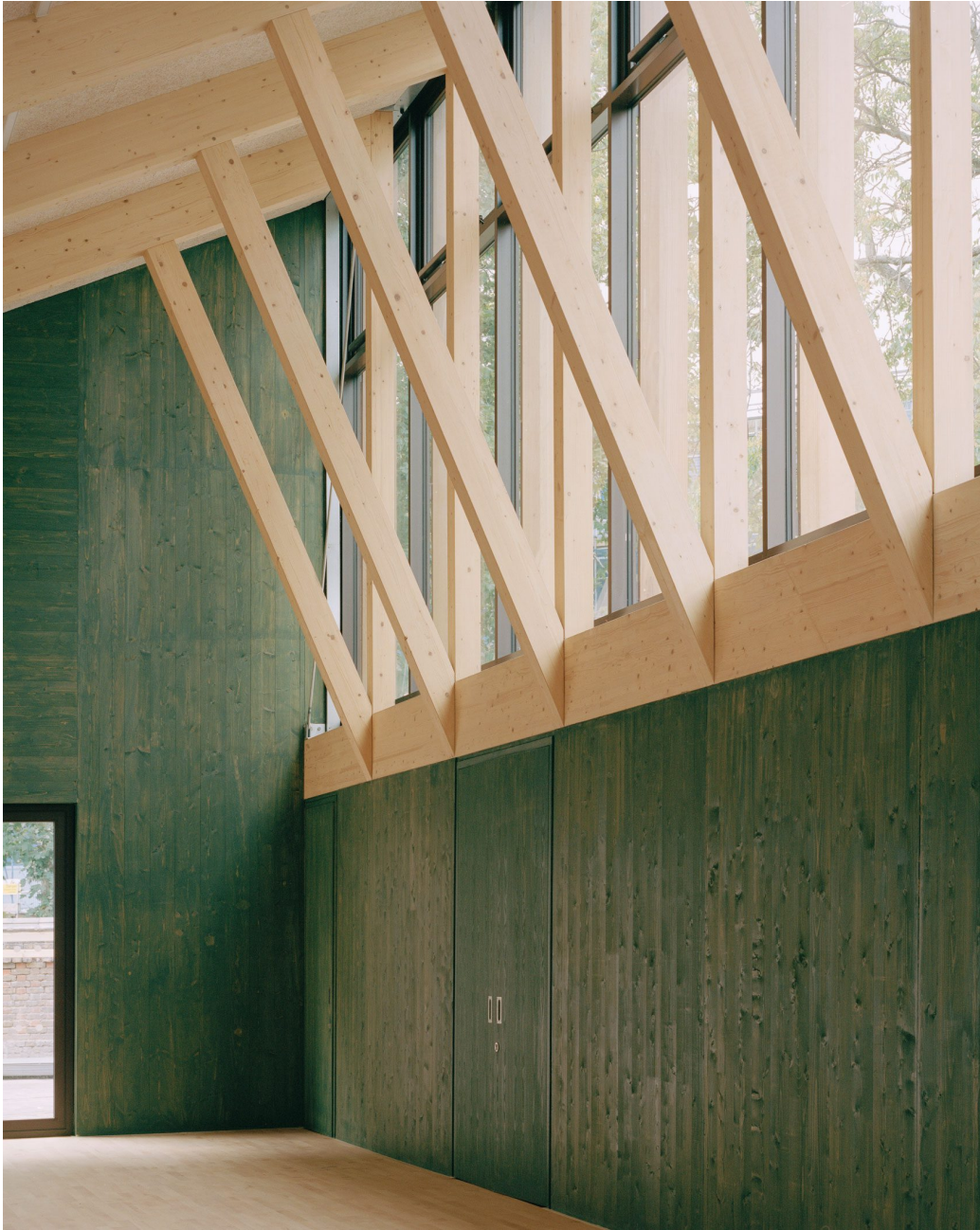
The cross-laminated timber structure of Mæ Architects' Sands End Arts & Community Centre in London. Credit: Rory Gardiner
