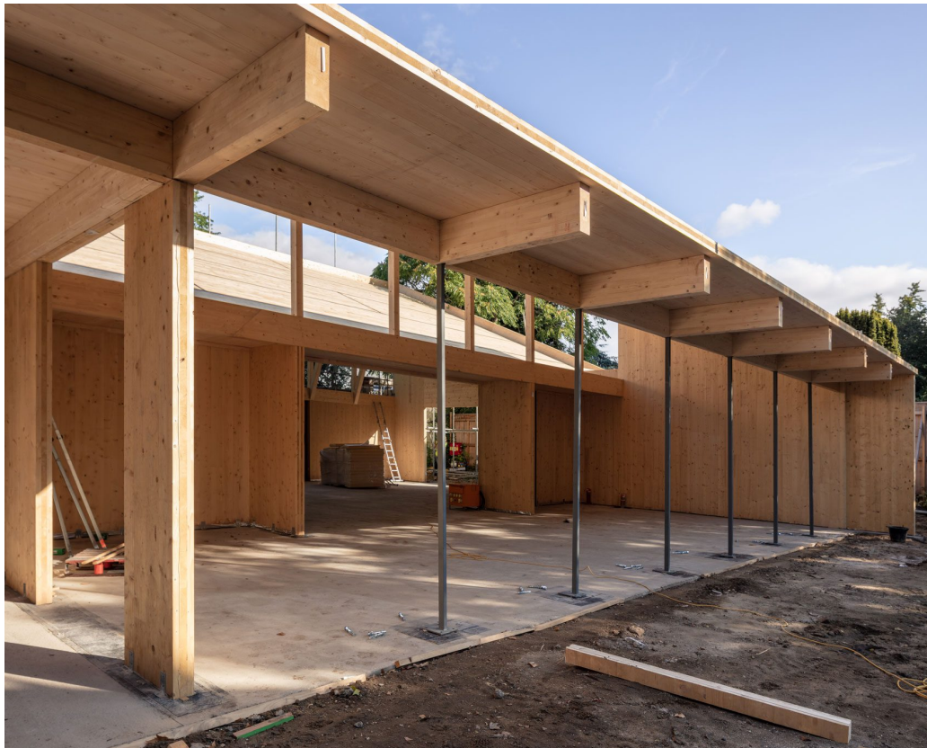
The cross-laminated timber structure of Mæ Architects' Sands End Arts & Community Centre in London has been designed to enable future disassembly. Credit: James Retief
